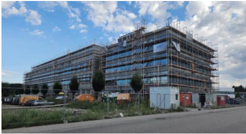
Freiburg, Germany Cell culture components
