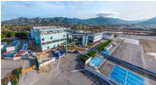
Aubagne, France Clean rooms, product development, labs
